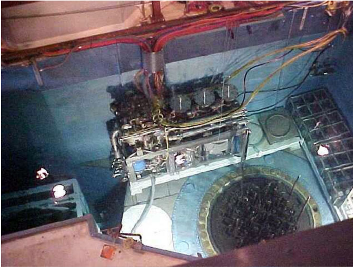
Backwash filtration for reactor vessel internals segmentation
