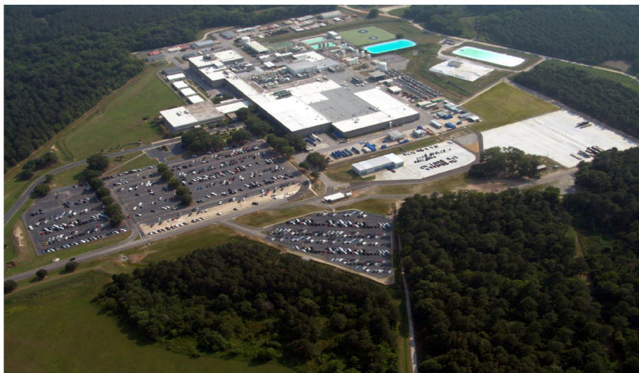
29 30 Figure 3-22 Aerial View of the CFFF Site and Facilities (WEC 2012-TN6697)
